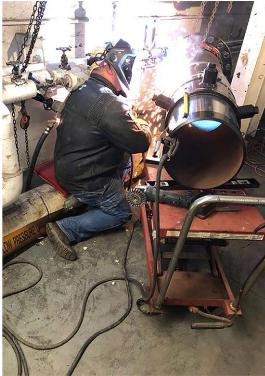
Steamfitter Durante is welding flanges to make final connections in a major repair to the steam-distribution line.
