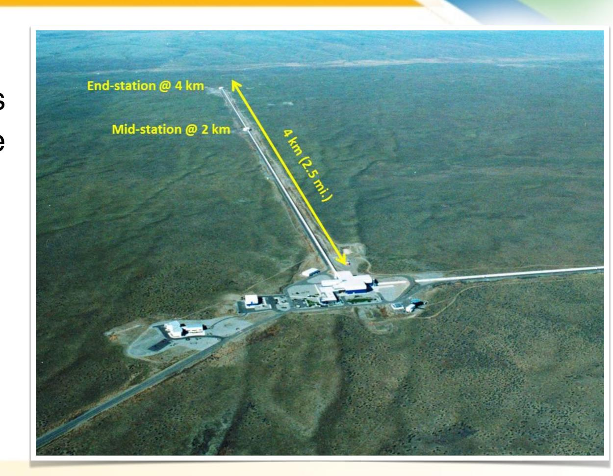
By measuring the interference of the lasers as they bounced between the different points we can measure very precisely whether the space in between has stretched or
